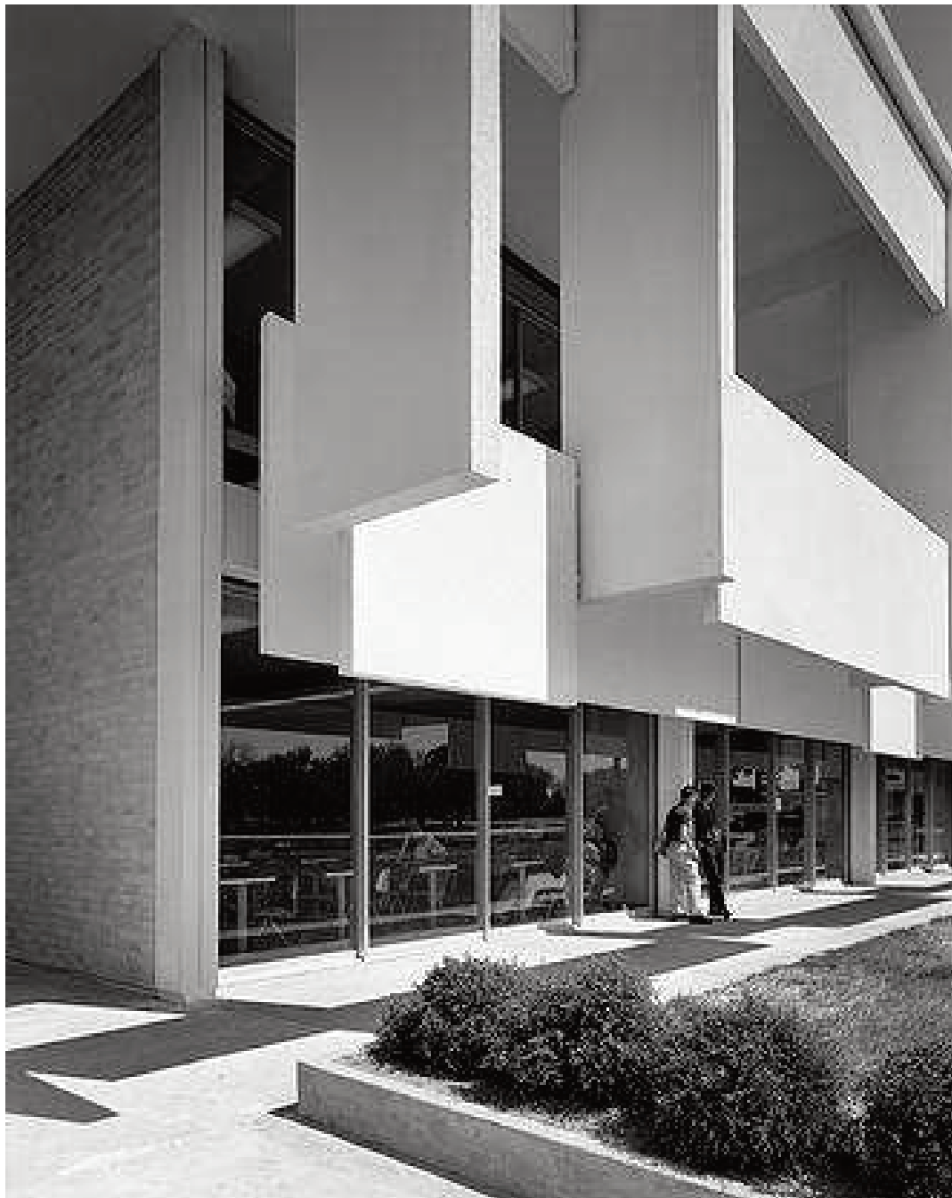
Sun shade detail, south side of classroom building no. 4
